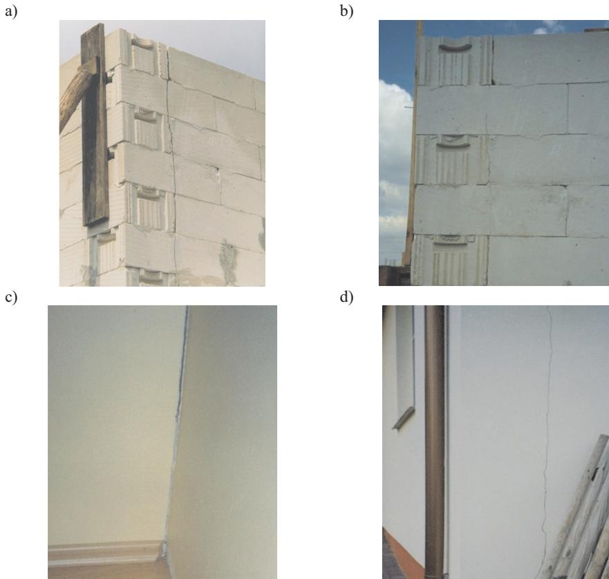
Fig. 2. Examples of cracks in walls corners (description in the text)
