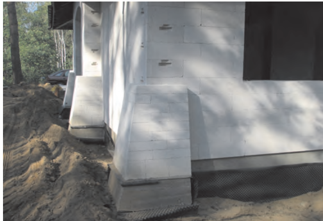
Photo 13. Detail in a uniform ACC wall made of precisely cut blocks. No other material can equal ACC
