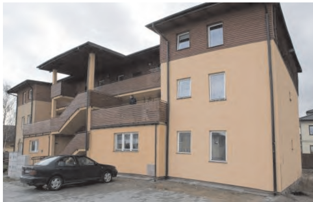
Photo 17. Building built by Habitat for Humanity using ACC located in Warsaw
