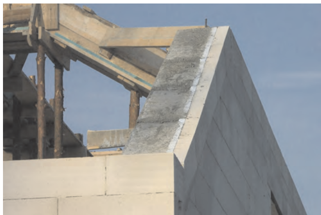
Photo 14. ACC wall can be fitted to every shape
