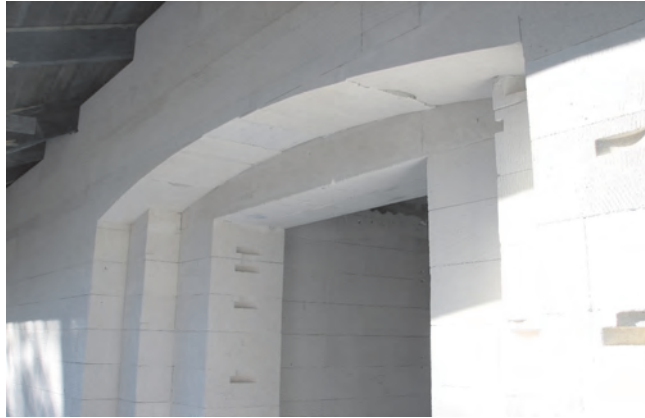
Photo 12. ACC enables making any given shape
