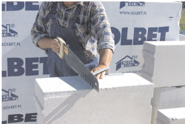
Photo 2. ACC elements are very easy to cut
