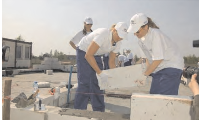
Photo 16. „Women build” campaign by Habitat for Humanity
