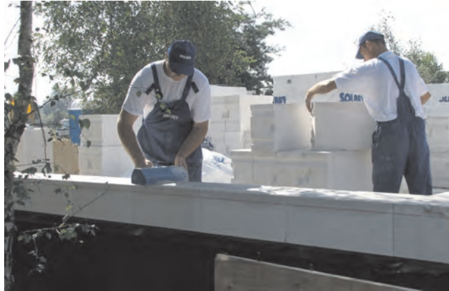
Photo 7. Thin layer bricklaying is very easy to perform
