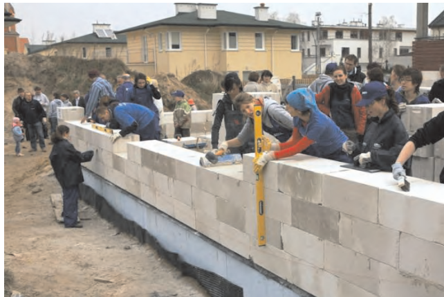
Photo 15. Building being erected by Habitat for Humanity
