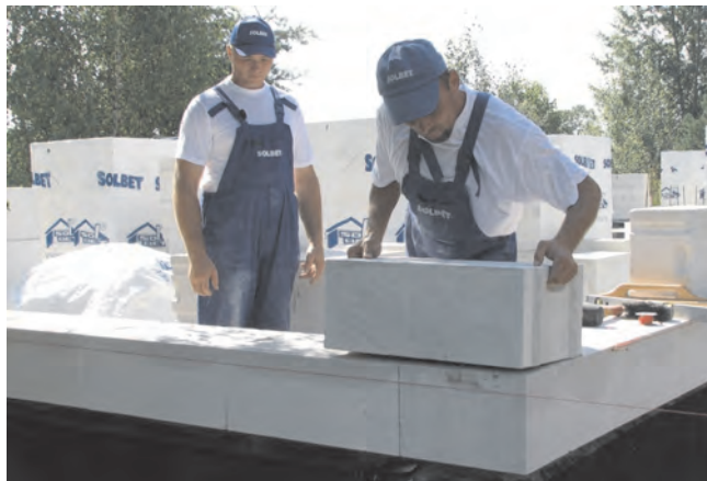
Photo 8. Precisely manufactured wall elements perfectly fit to one another
