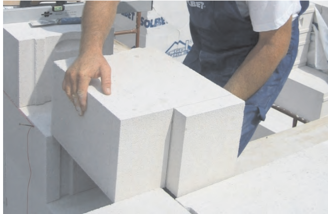
Photo 3. Blocks can be easily cut and fitted to every shape
