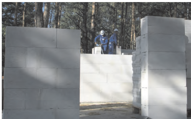
Photo 4. Small weight enables manufacture of large and ergonomic ACC wall elements
