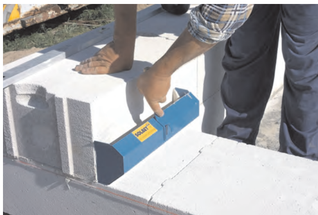
Photo 6. It is necessary to use basic tools for thin layer bricklaying
