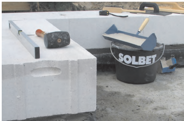
Photo 5. Basic tools for ACC system bricklaying
