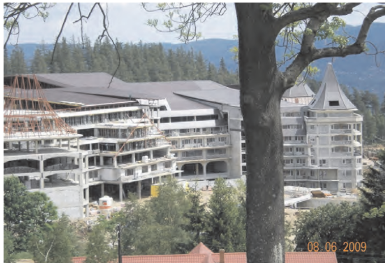
Photo 9. Gołębiewski Hotel in Karpacz. Reinforced concrete structured filled with ACC wall elements
