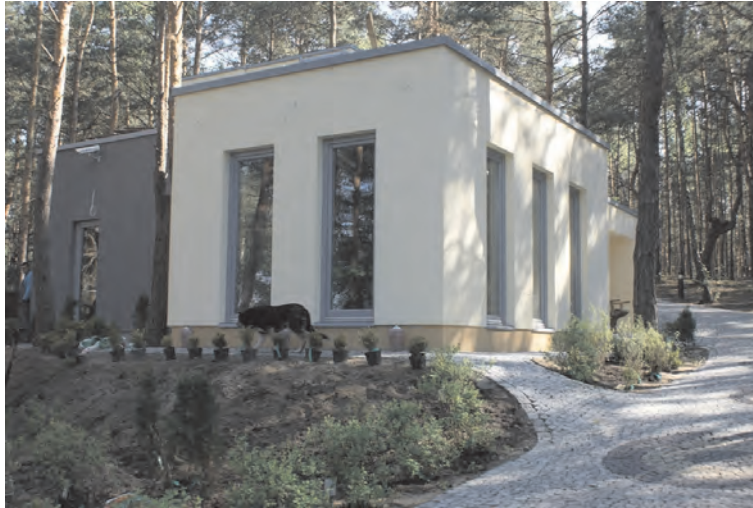
Photo 3. Passive building of ACC construction
