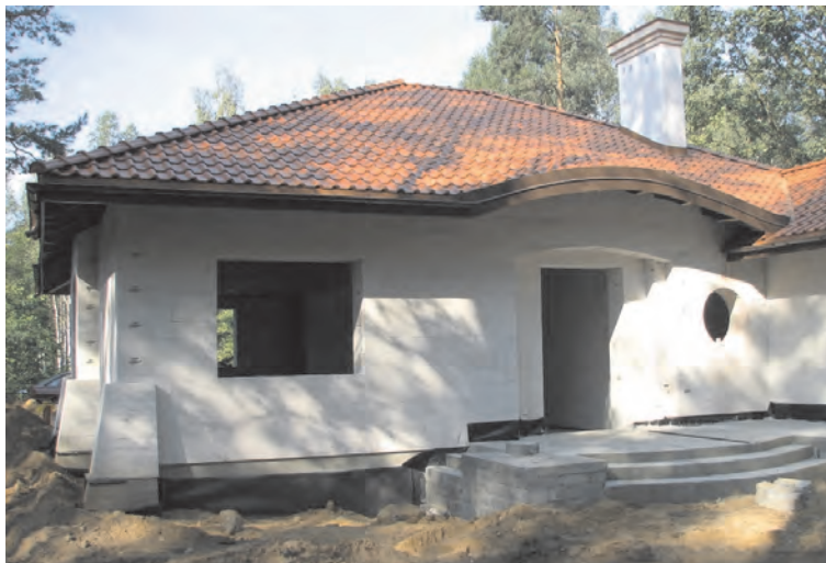
Photo 2. Single-family building of ACC construction, system-based project by a small construction company
