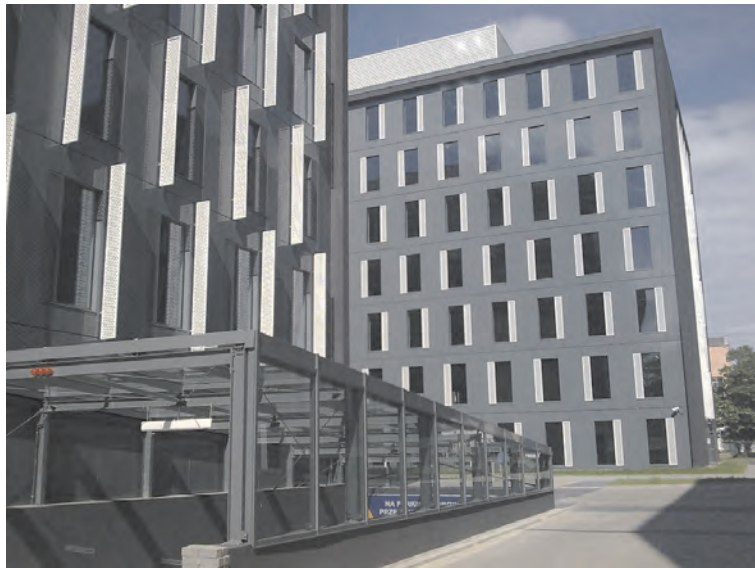
Photo 11. Office building with ACC infill walls
