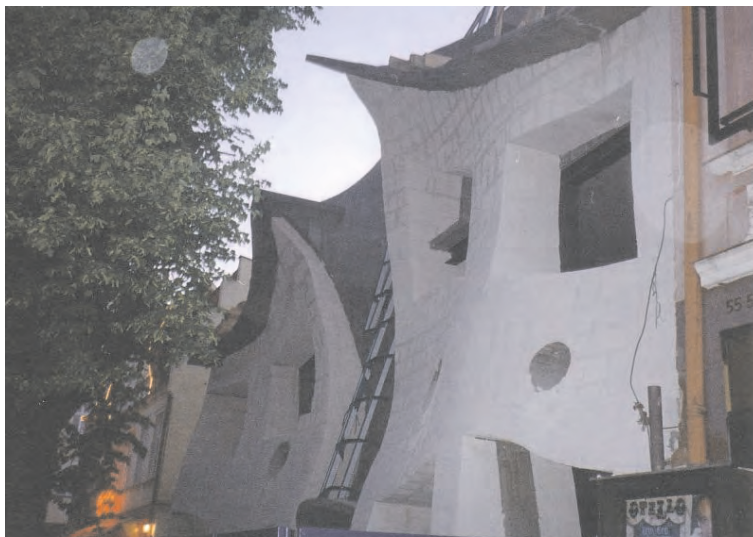
Photo 4. The Crooked House in Sopot under construction. Front made of ACC.
